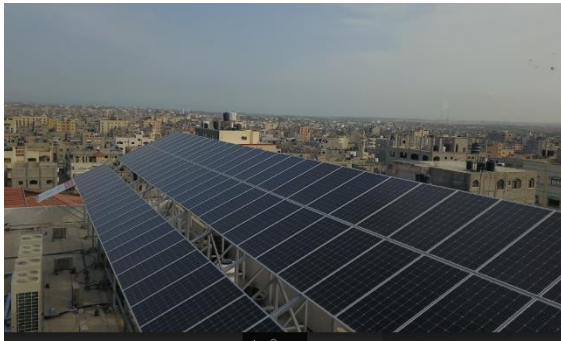
Example of Roof and Façade Mounted Solar Panels (Islamic University of Gaza)
